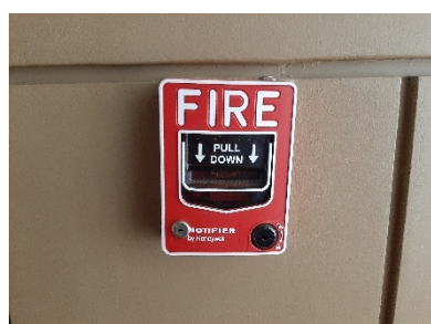
fire alarm manual station
