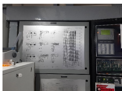
Graphic Annunciator Fire Alarm System
